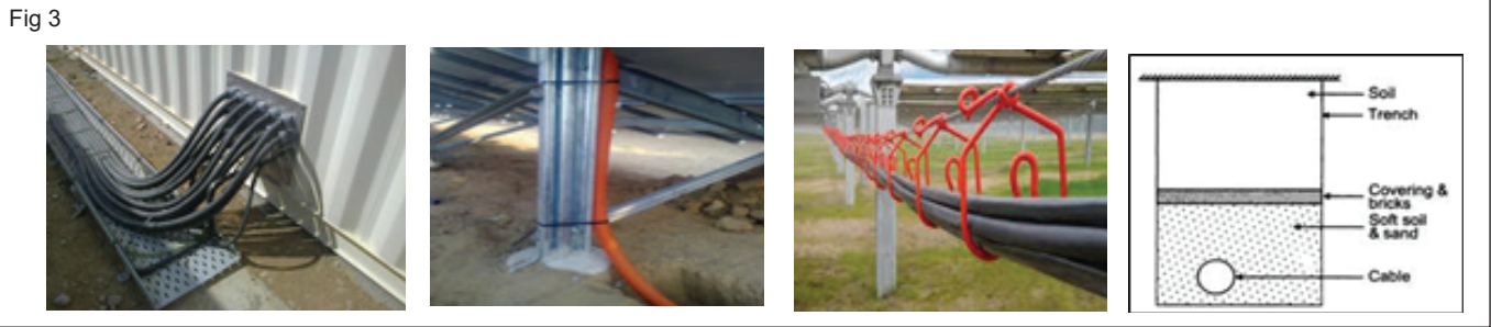
Fig 3 Cable laying and extension
