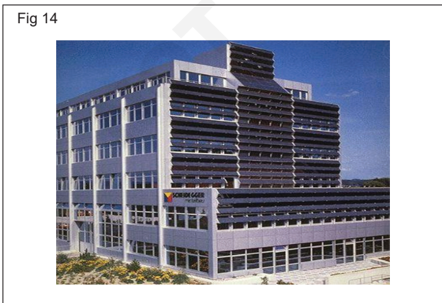
Fig 14 Building with Photovoltaic Façade
